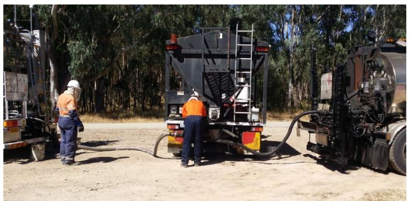
**Fig 1** Field blending and transfer of crumb rubber polymer modified binder using bulk blending unit
