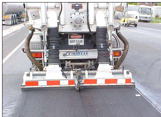
Figure 1 Surface Cleaning Machine with Truck Mounted Cutting Heads
