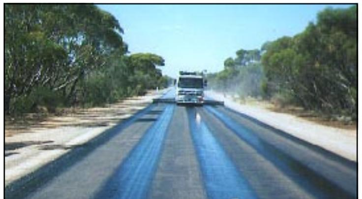
Figure 3 Applying final spray
