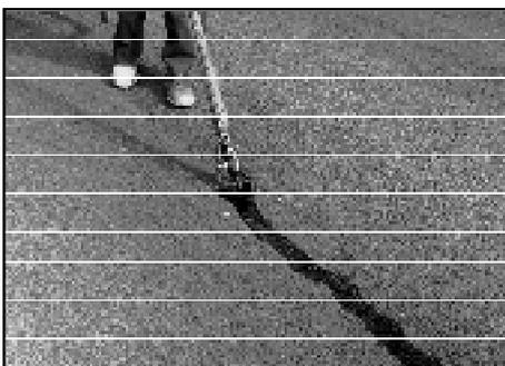
Crack filling with insulated hand lance
