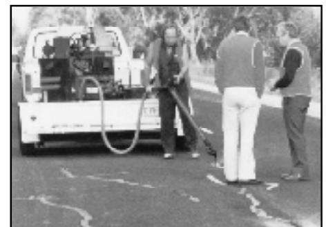
Filling and sanding cracks after routing
