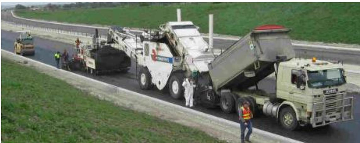
Asphalt paving with a Materials Transfer Vehicle.
